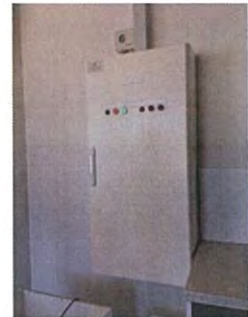
Heating/Cooling Unit Fuse Box
