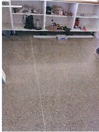
Kitchen Area and Kitchen Flooring- Polished Concrete
