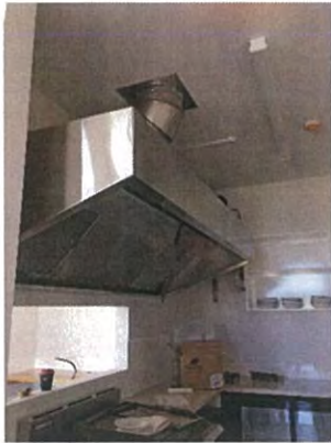
Extraction Hood - Stainless Steel
