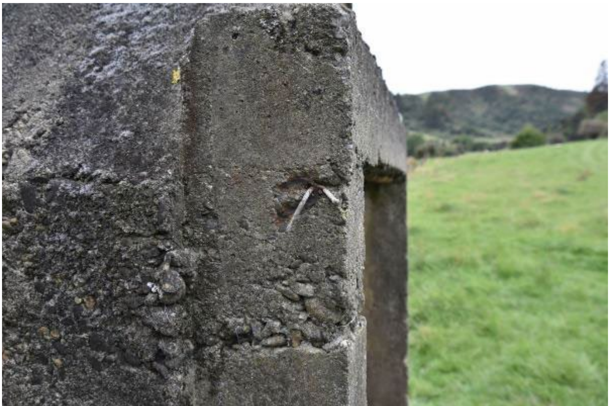
Photo 6 Galvanised steel wire nail attached to the steel rod lintel (likely post 1945).
