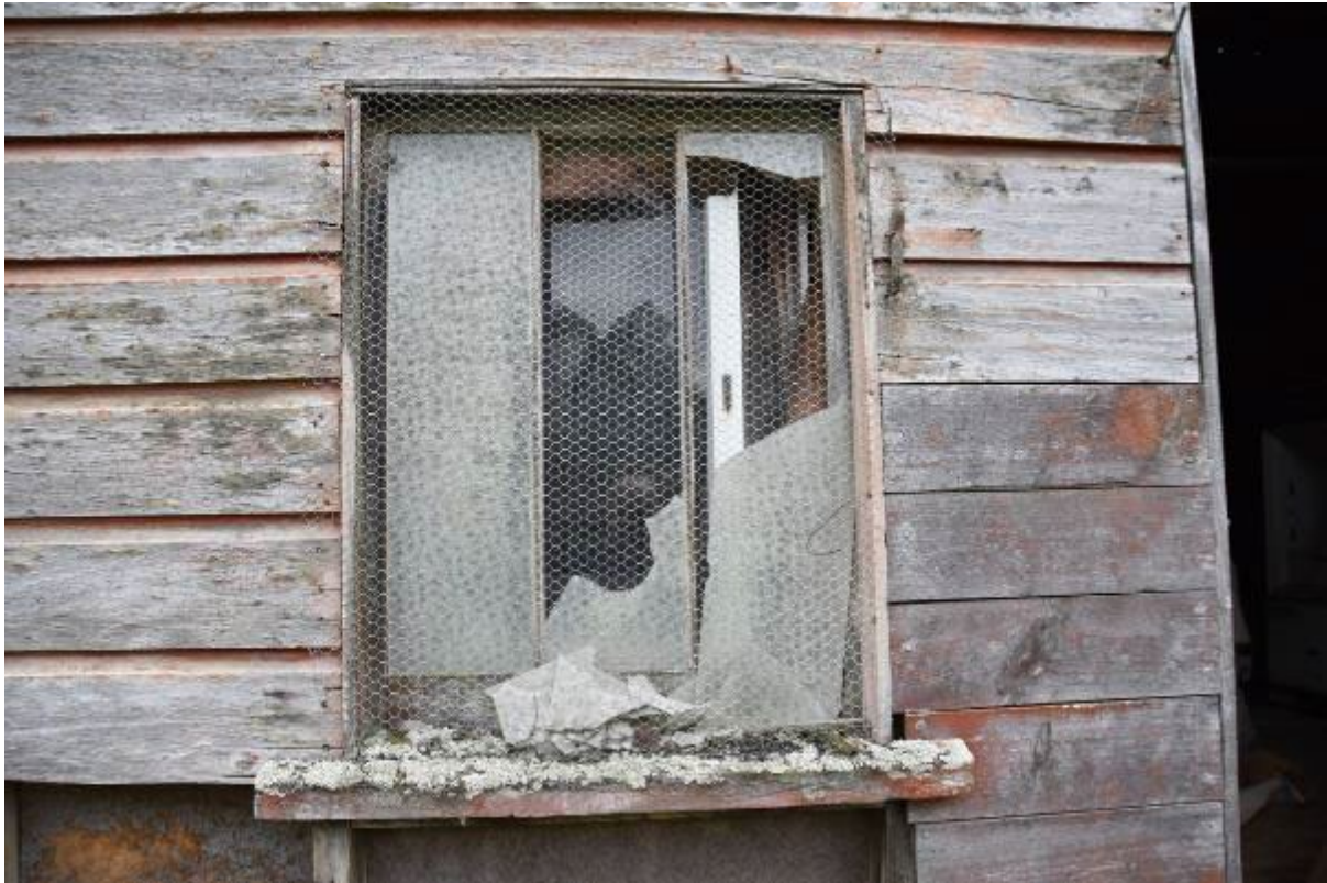
Photo 23 The other three-light ground floor south elevation window (with pressed pattern glazing).
