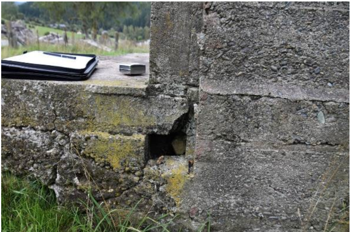
Photo 2 Bottom plate pocket for a framed wall with the rusticated weatherboard line adjacent on the right.
