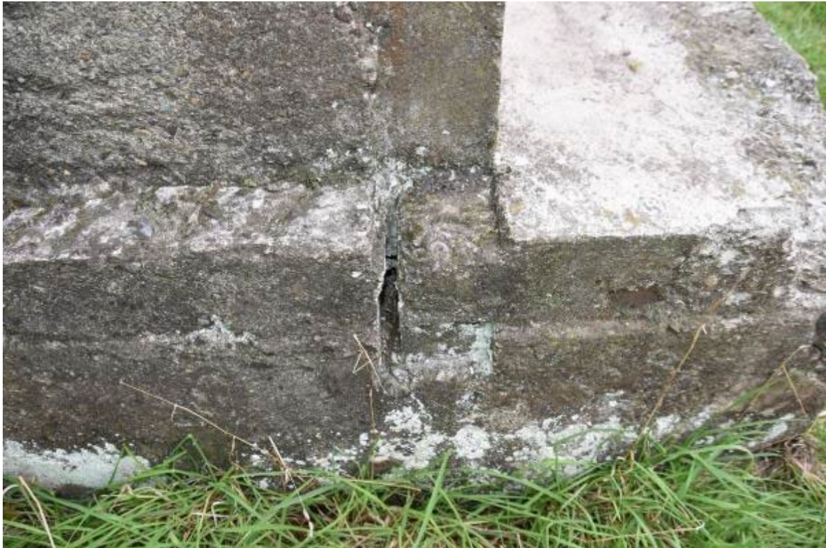
Photo 9 Bottom plate and weatherboard imprint in the concrete on the other side of the chimney to that shown in photo 2.
