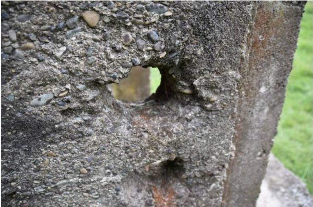
Photo 7 Holes in the side of the fireplace likely to be for pipework (wetback, etc). Wire reinforcing exposed in the holes.
