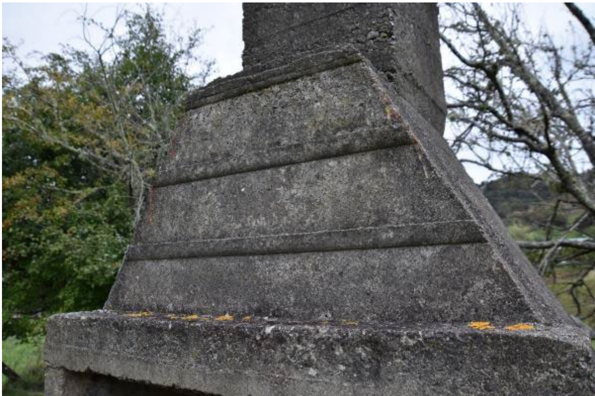
Photo 4 Rusticated weatherboard imprints in the concrete above mantel level.
