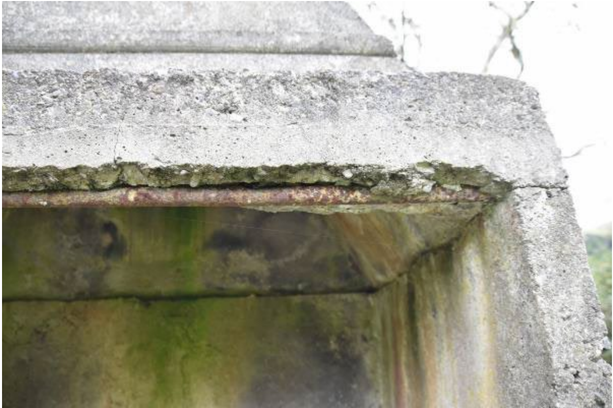
Photo 5 Hollow steel rod cast into the concrete to act as a lintel over the fireplace opening.
