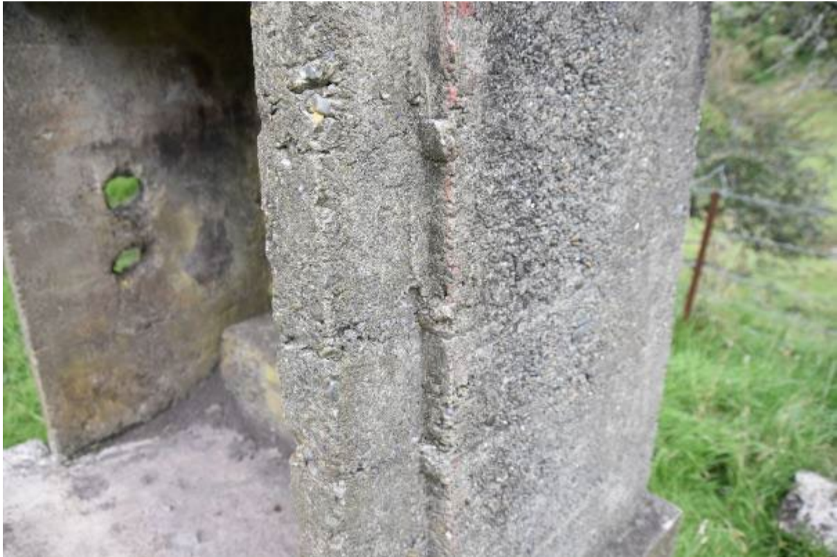
Photo 3 Rusticated weatherboard imprints where the concrete was cast against them.
