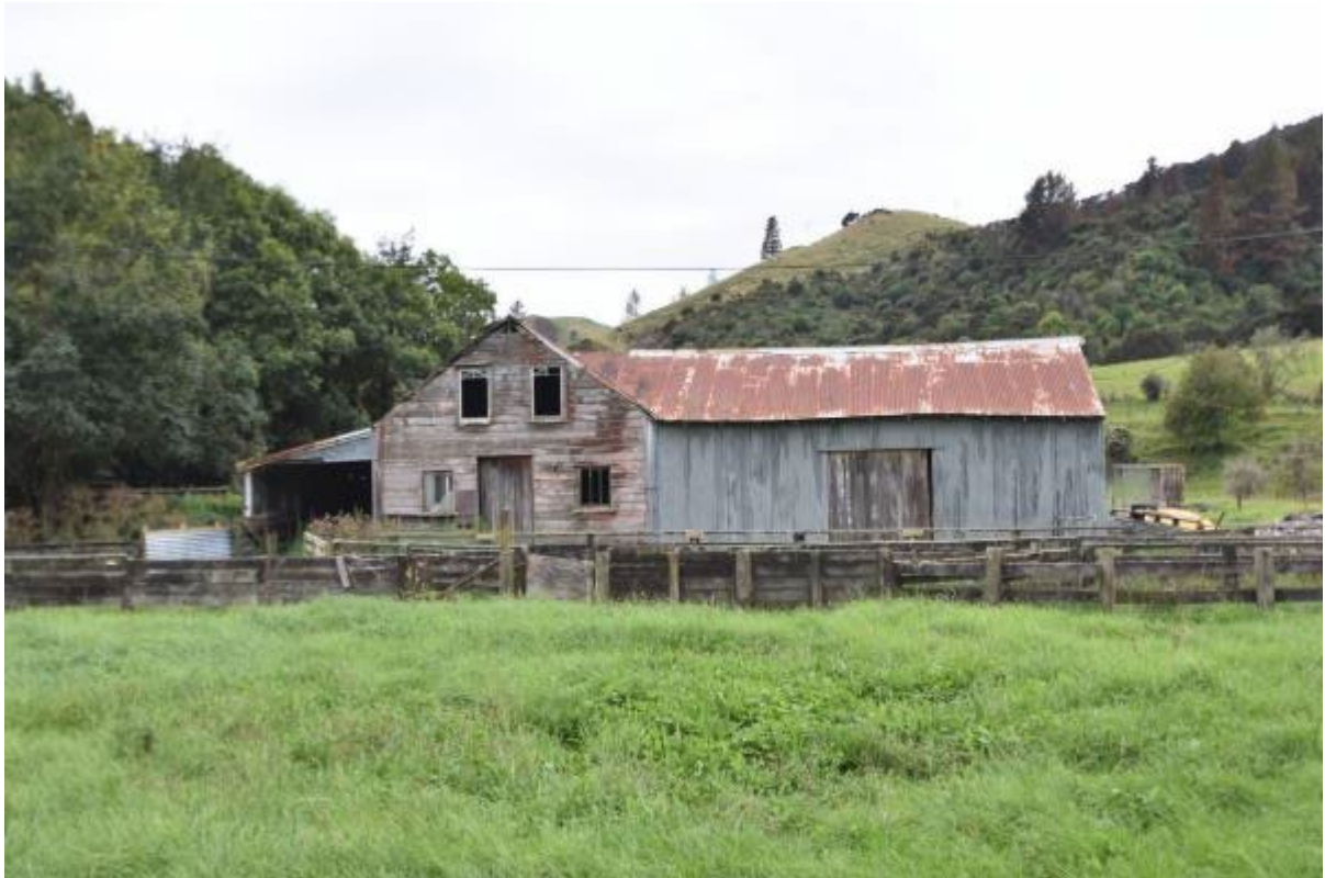
Photo 15 The south elevation with the timber weatherboard-clad gable to Building Part A. Building Part B is the corrugated iron-clad addition on the right. The lean-to on the left is Building Part C.
