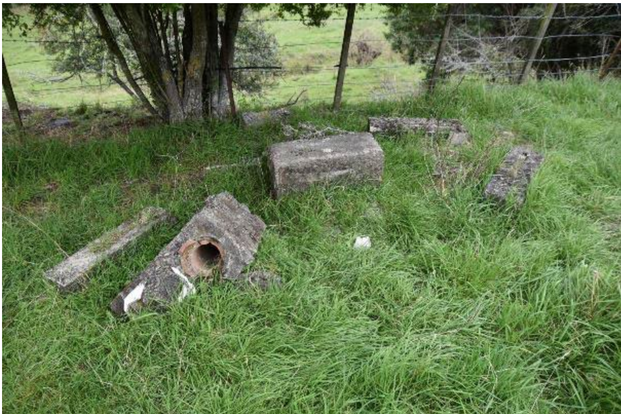
Photo 14 Concrete rubble incorporating the base of a white ceramic sanitary fitting and a sewer pipe.
