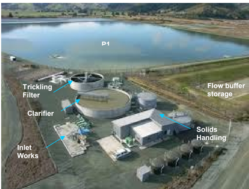
Figure 2: Aerial photograph showing key components of NWWTP Pre-treatment Plant (P1 in background)
