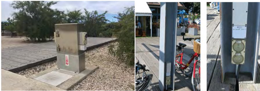
Above: Standalone and part of a structure power supply boxes
